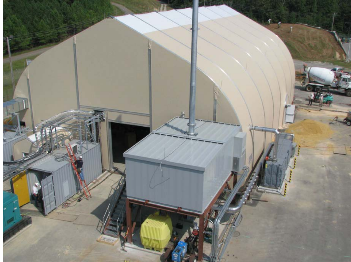
Shown is the Anniston SDC Facility
